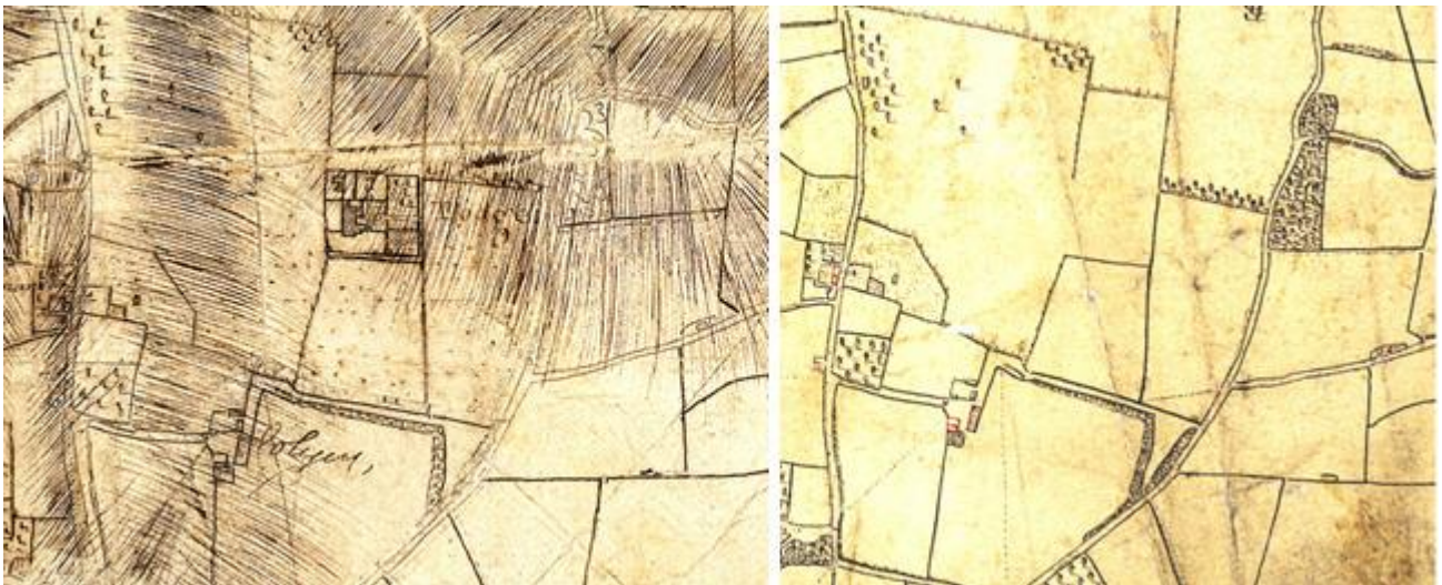
Figure 4 Teynham Lodge (a) on trace (ser 431) and (b) as a gap on OP (ser 433)
