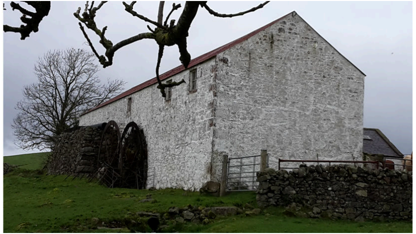
Figure 5: Left: OS first edition 25-inch mapping of Chapel farm near Dunscore showing the mill dam and sluice, with the lade (single line) leading to the unrepresented overshot water wheel and unlabelled threshing barn (above right). The water wheel is connected through the wall of the barn to the thrasher inside the barn (right). The sheaves were fed into the rollers at middle left and threshed in the lower drum, and elevated to the upper drum where the grain was winnowed. The lade at Chapel is piped and the second edition 25-inch mapping has a diagrammatic representation of the water wheel. 6
